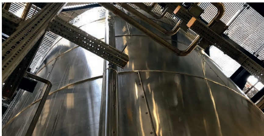
These 85,000 litre fermenters in Leuna, Germany, are making bio-1,3-butylene glycol
