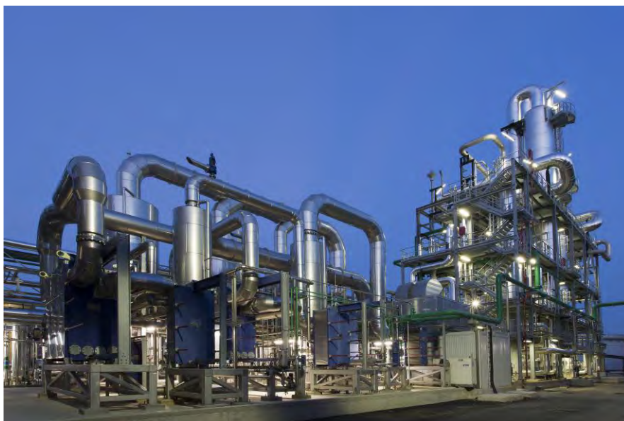
Novamont has opened the world's first commercial-scale plant for the bio-based production of a major intermediate chemical. Using Genomatica's GENO BDO™ process, it will produce 30,000 tons of BDO per year from renewable sources rather than fossil fuels.
